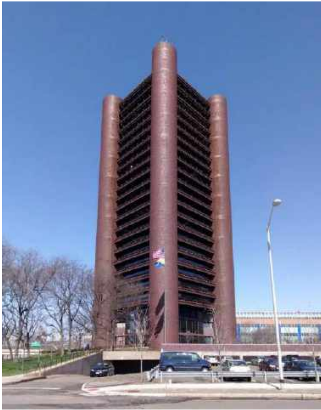
Figure: Knights of Columbus Building, New-Haven, Connecticut
