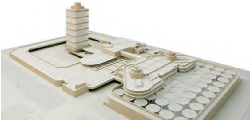
Figure: Johnson Wax Building by Frank Lloyd Wright. Mushroom column can be seen under the glass floor.
