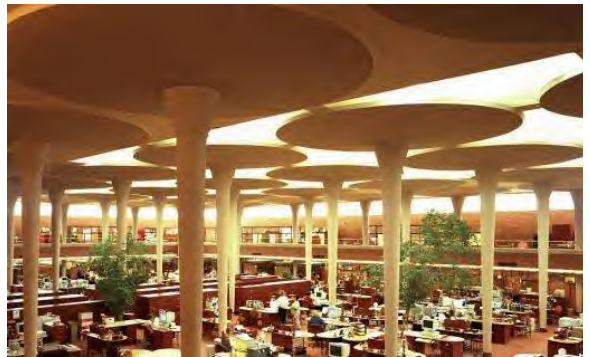
Figure: Inside view. Johnson Wax Building by Frank Lloyd Wright. Mushroom column.
