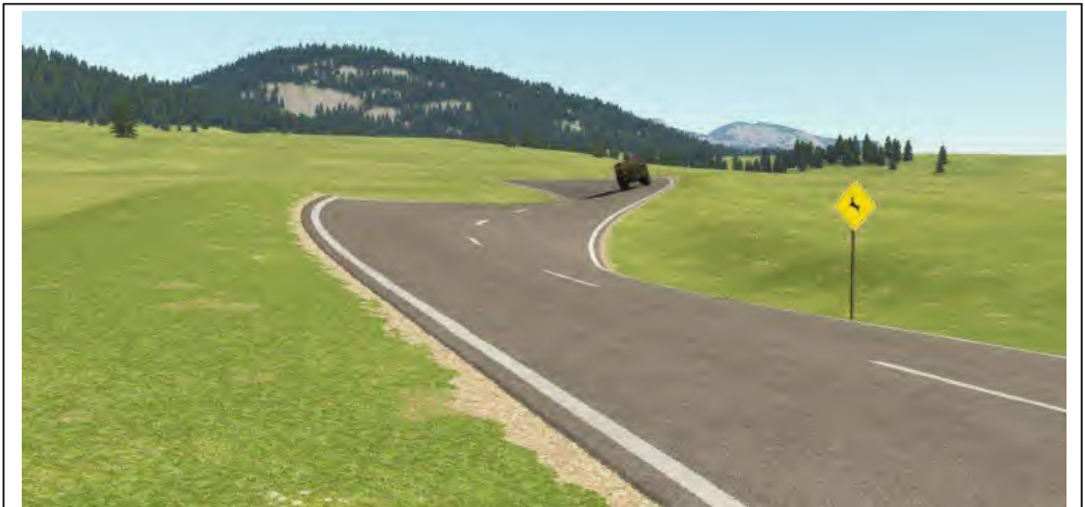
Figure: Super elevation is tilting the roadway to help offset centripetal forces developed as the vehicle goes around a curve. Along with friction they are what keeps a vehicle from going off the road.
