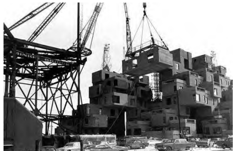
Figure: 354 prefabricated individual containers are stacked in a confused order and connected by steel cables.
