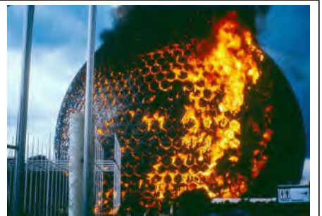
Figure: The sphere would remain open to the public for nine years until an accident involving some routine welding maintenance caused the acrylic covering to catch fire, engulfing the entire sphere in a spectacular ball of fire with flames that burned for 30 minutes. When the flames subsided, there was no sign of the acrylic walls to be seen, but the steel trusses of the dome remained. After the fire, the dome was closed to the public for over fifteen years. (Photo credit - collectionscanada )
