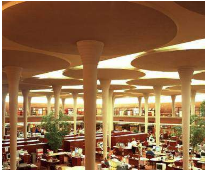
Figure: Inside view. Johnson Wax Building by Frank Lloyd Wright. Mushroom column.
