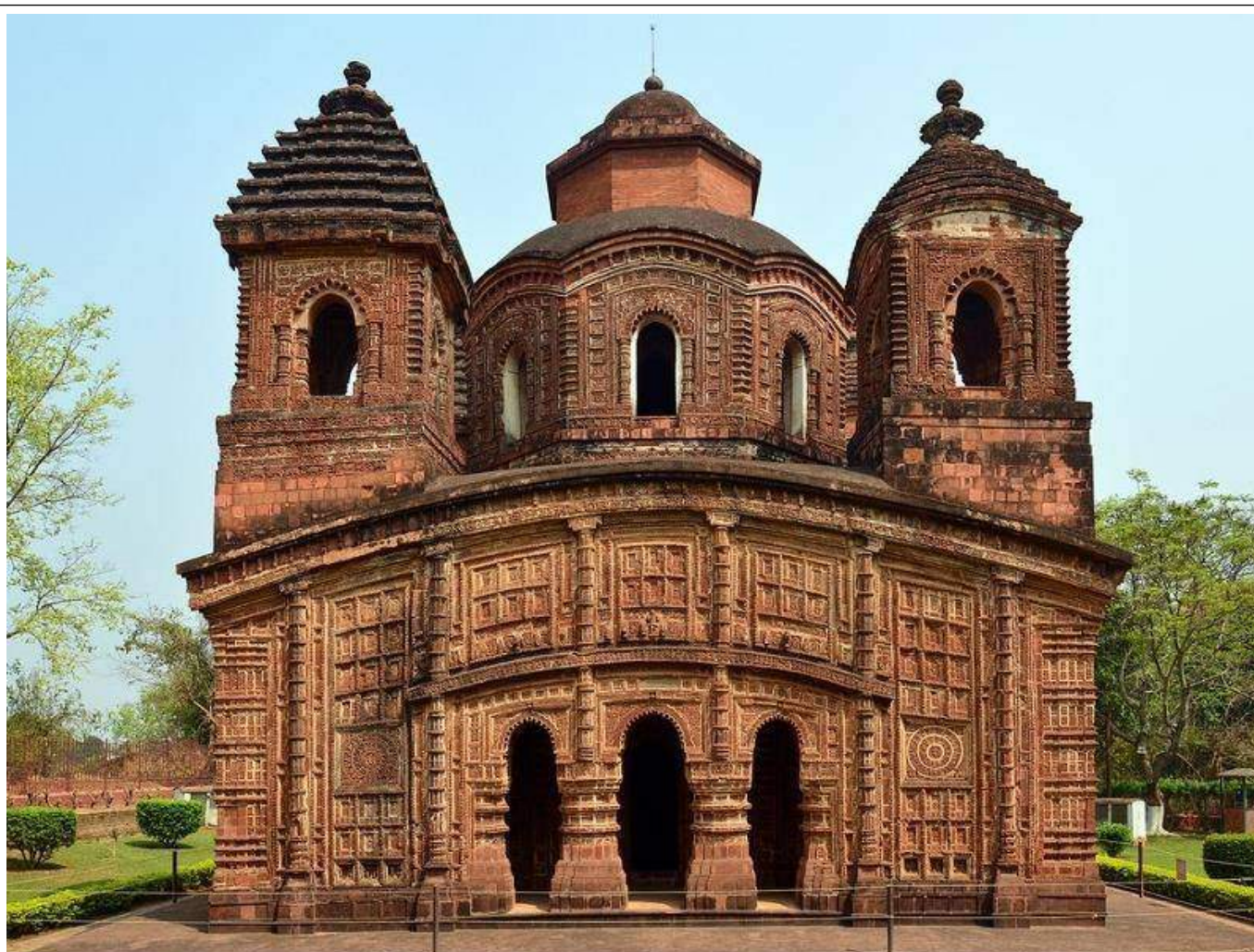
Figure: Shyam Rai Temple, Bishnupur, West Bengal. It is built in the Panchratna Architectural style (in which five pillars stand on the roof). Four pillar stands an four corners and one at the centre. The word Panchratna means Panch = five & Ratna = Gems.
