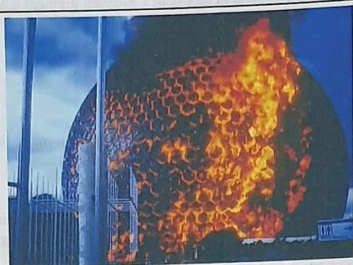
Figure: The sphere would remain open to the public for nine years until an accident involving some routine welding maintenance caused the acrylic covering to catch fire, engulfing the entire sphere in a spectacular ball of fire with flames that burned for 30 minutes. When the flames subsided, there was no sign of the acrylic walls to be seen, but the steel trusses of the dome remained. After the fire, the dome was closed to the public for over fifteen years. (Photo credit - collectionscanada )
