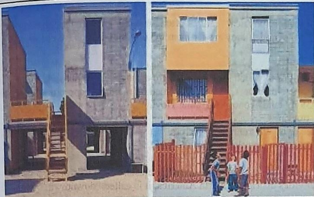
Figure: There are two photographs here. Aravena provided a concrete frame, with kitchen, bathroom and a roof (left), which were designed to allow families to fill in the gaps (right). So, the architect provided a basic concrete frame, complete with kitchen, bathroom and a roof, allowing families to fill in the gaps, and stamp their own identity on their homes in the process. Photograph: Cristobal Palma, Source: www.theguardian.com
