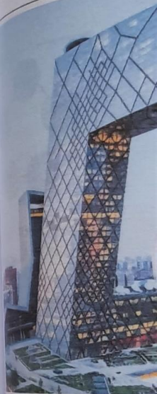
GATE 2006: Koolhaas reinvented the office building as a vertical city, the headquarters for CCTV. The building is connected by a 246-foot cantilevered overhang. The exterior is a striking pattern of triangles, and the support structure is a series of columns.
