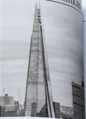
ard building, London by Renzo used gives the building a lightness
