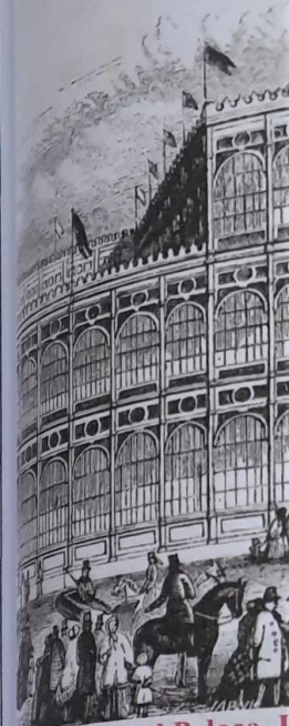
GATE 2015: Crystal Palace, I prefabricated parts. It consisted the building was 1,848 feet (563 m aces). The construction occupied at 92,000 square metres, or abo of display tables.
