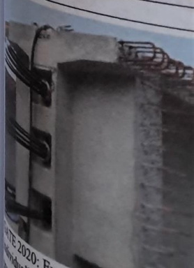
GATE 2020: Example of post tensioning. Image shows a tendon in a concrete slab.
