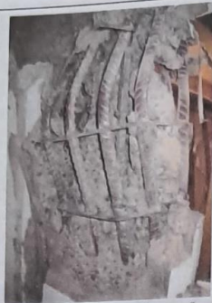
GATE 2020: Buckling of Concrete Columns.
