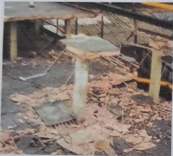
GATE 2020: Flat Slab Failure due to Punching shear.
