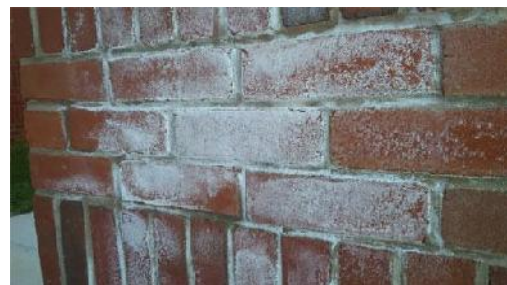
Figure: Efflorescence is the migration of a salt to the surface of a porous material, where it forms a coating. The essential process involves the dissolving of an internally held salt in water, or occasionally in another solvent. The water, with the salt now held in solution, migrates to the surface, and then evaporates, leaving a coating of the salt.
